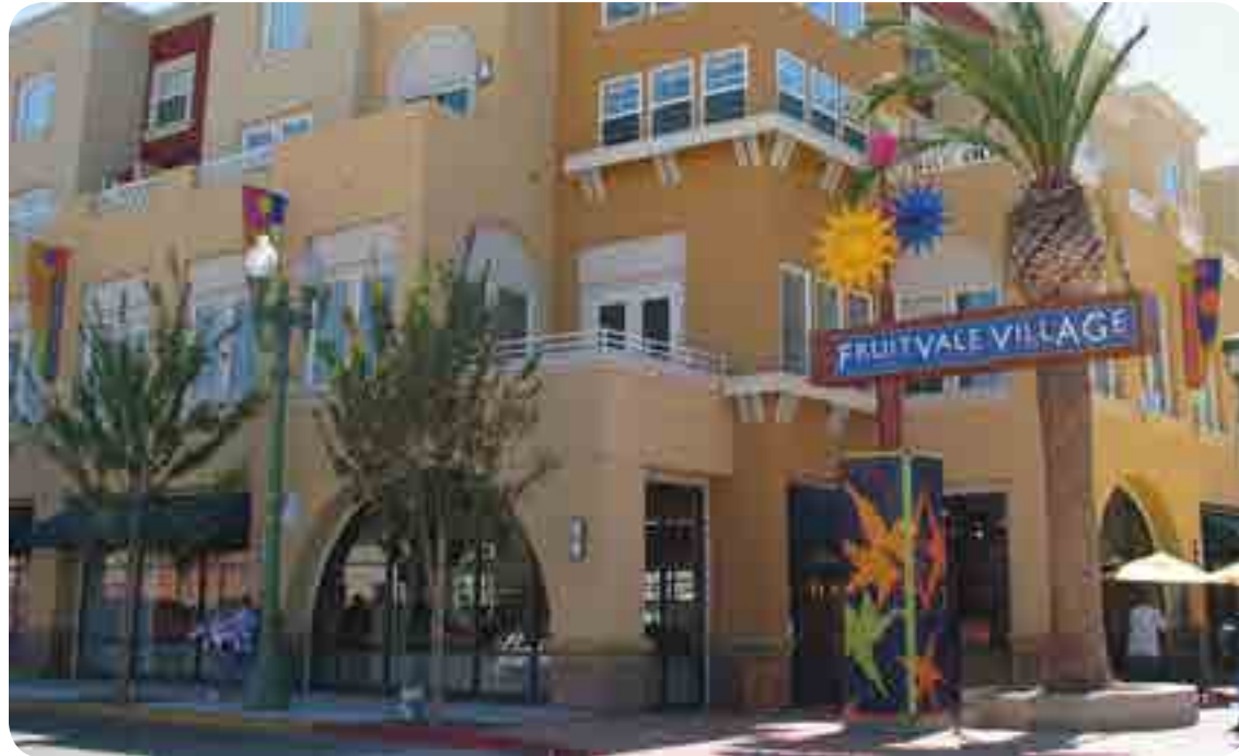
Fruitvale Village represent transit-oriented development that connects with the neighborhood through culture, housing, retail and community resources. Square Peg Design. Photo: BART
