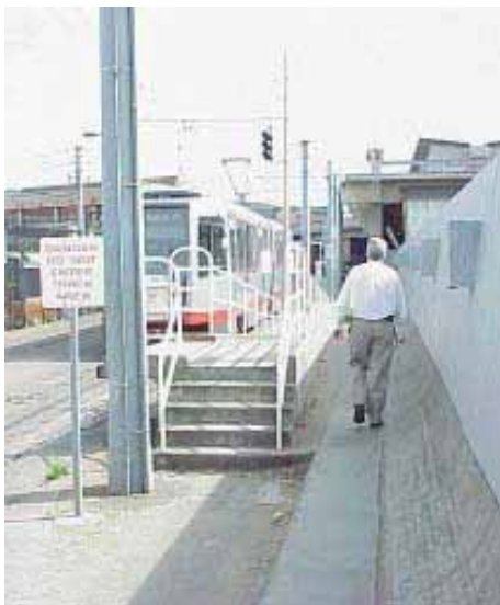
The new pathway would replace the informal route alongside the Muni streetcar tracks.
