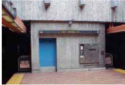
Should a passenger follow the sign for the emergency stair, or obey the 'Danger: Electric Third Rail. Do not Enter' sign?
