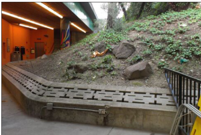
Site of recommended retaining wall, stairs and inverted “U” racks
