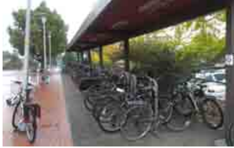
Site of recommended double deck rack system
