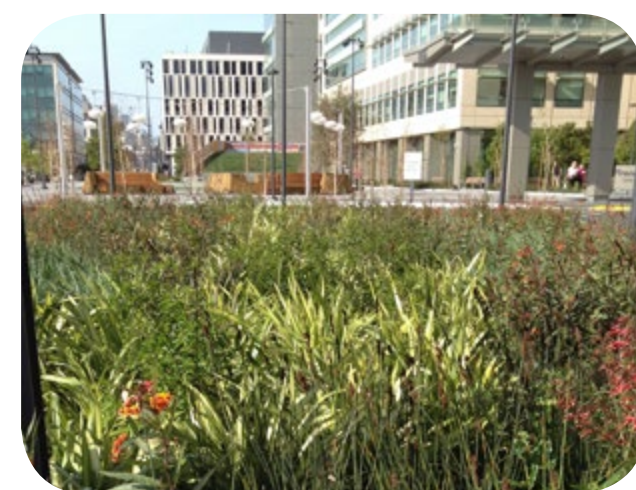
Bio-swale at UCSF Mission Bay
