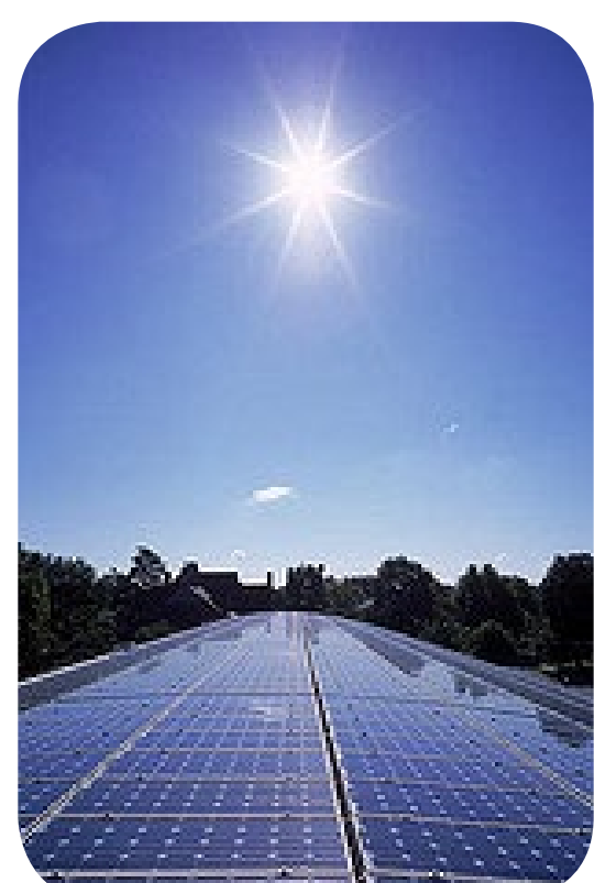
Solar panel array
