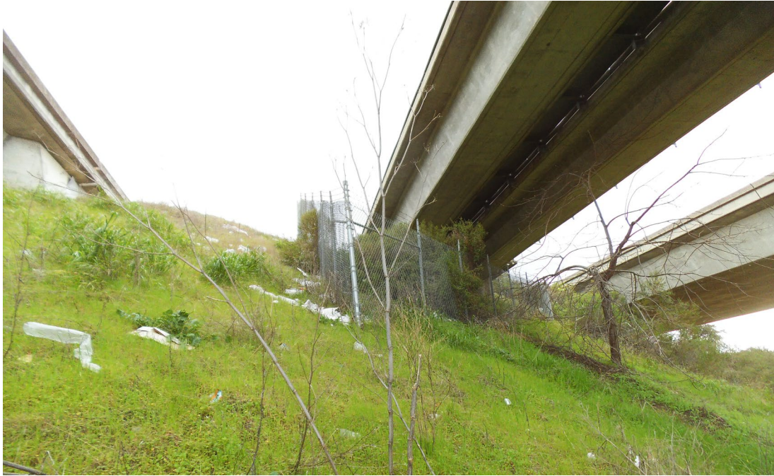
Note: Project site is the middle structure and the slope below, as viewed from Kinne Blvd., looking east. Figure 9. View of Concord Project Site C3015E
