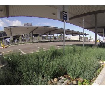
10,820 square feet of LID were installed, ensuring the stormwater runoff from each site is captured and treated
