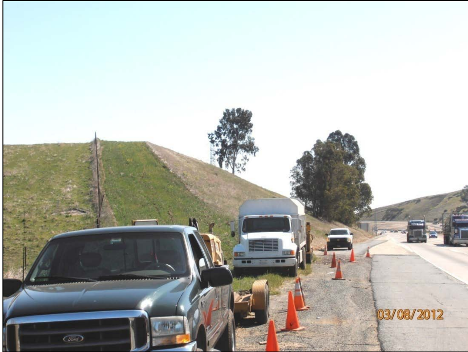
Photo 1: View of Knoll looking east from shoulder of SR 4
