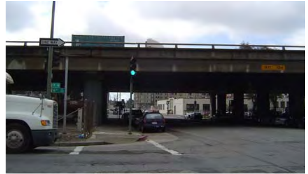
Freeway underpass at 6 th and Oak
